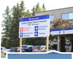
Bulkley Valley District Hospital – Smithers
