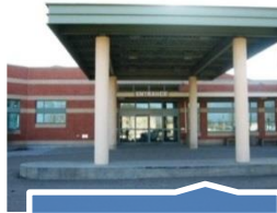
Dawson Creek and District Hospital
