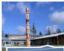
Haida Gwaii Hospital and Health Centre
