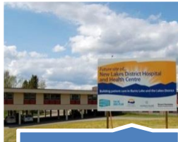
Lakes District Hospital – Burns Lake
