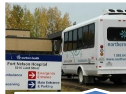
Fort Nelson Hospital
