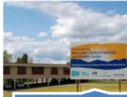
Lakes District Hospital – Burns Lake
