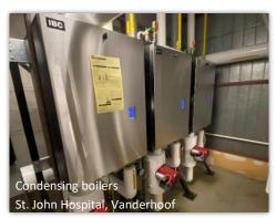
St. John Hospital in Vanderhoof received five new condensing boilers in 2019 along with pumps, piping and duct work to support heat recovery coils and reheat coils. In 2020 a new air to water heat pump was added to take heat from air handling exhaust, releasing heat into the low temperature heating loop for air handling pre heat coils. This allows the use of large natural gas boilers to be offloaded in low load and shoulder seasons.
