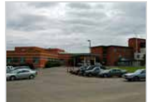
Dawson Creek and District Hospital
