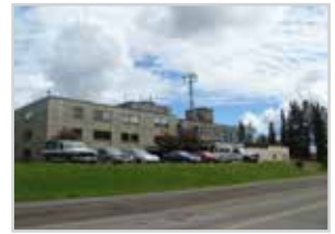
Bulkley Valley District Hospital, Smithers
