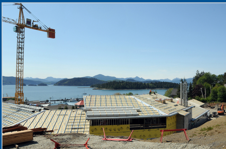
New Queen Charlotte Islands General Hospital (under construction)
