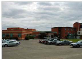
Dawson Creek and District Hospital
