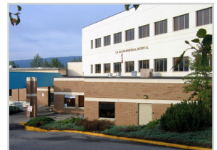
GR Baker Memorial Hospital, Quesnel
