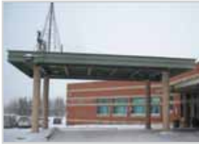
Dawson Creek and District Hospital
