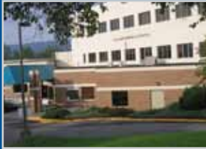
GR Baker Memorial Hospital, Quesnel
