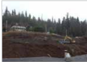
QCI General Hospital excavation
