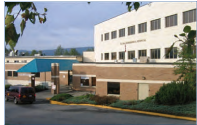
GR Baker Memorial Hospital, Quesnel
