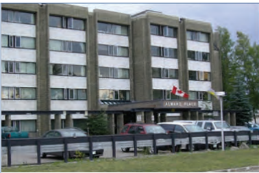
Alward Assisted Living Facility, Prince George
