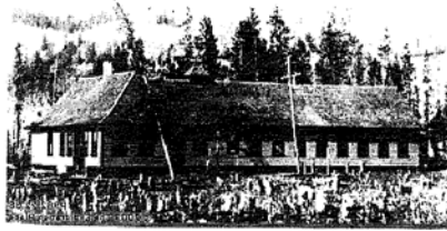
(Grand Trunk Railway Hospital)
