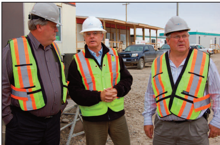
B.C.’s Minister Responsible for Housing, Rich Coleman (left), toured the hospital and residential care construction site on November 4, 2010, with Project Director Tom Sparrow (centre) and Pat Pimm (right), MLA for Peace River North.
