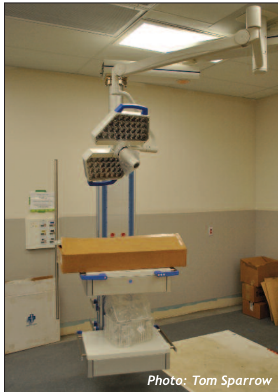
This trauma light and boom is one of the many pieces of equipment that will be extensively tested before being validated for use.
